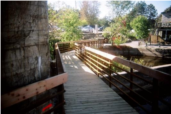
Riverwalk Bridges Opening Day 2005
